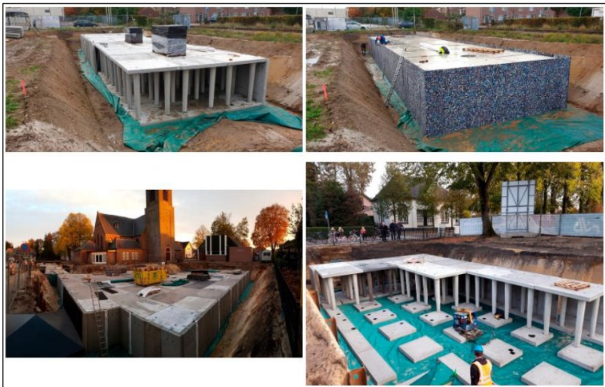
Figuur 5: Impressie Watertable-systeem (bron: www.trewatin.nl )
