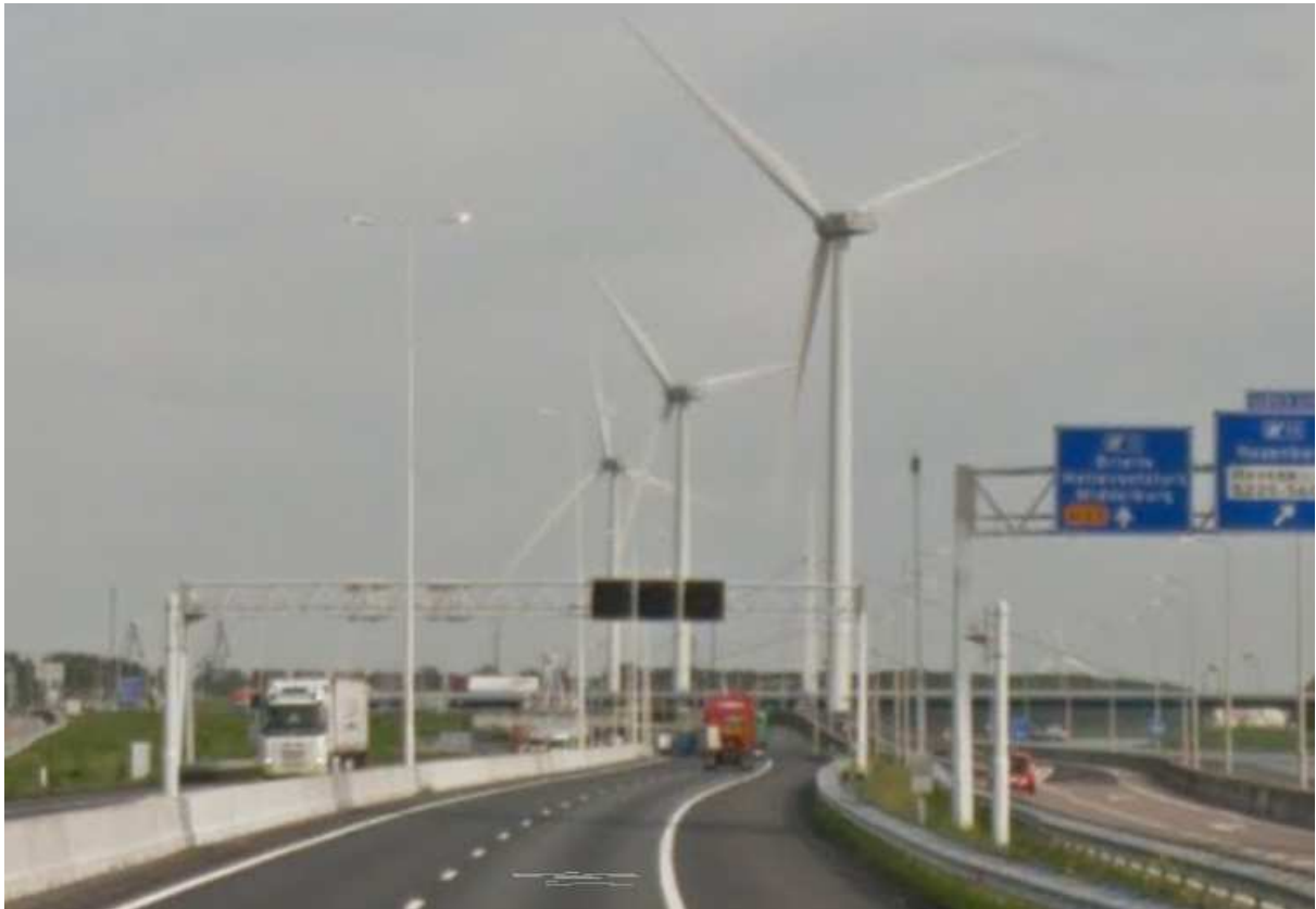
Afb. 6.6: De turbines langs de N15 (thans A15). Bron: Google Streetview.
