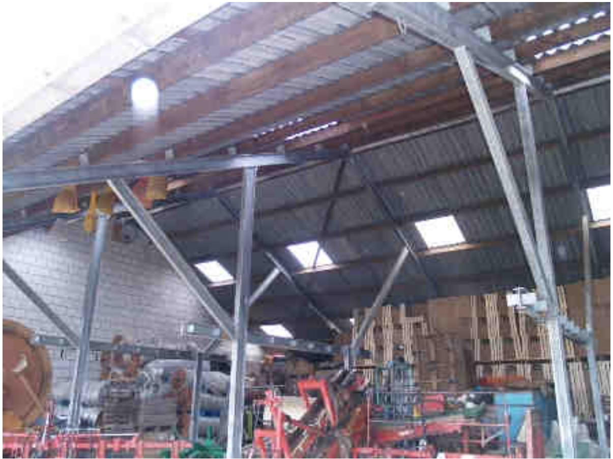
Te slopen stal
