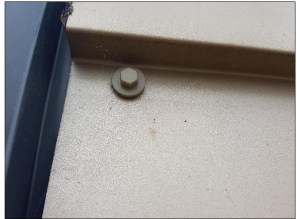
Figuur 6. Detail beplating hotel
