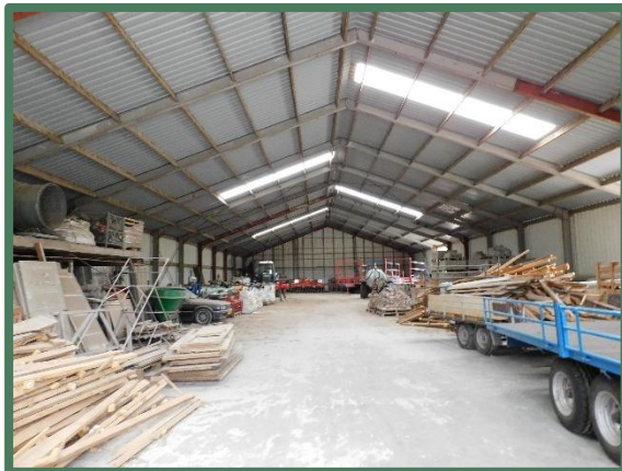
Foto 11: Binnenzijde halfopen loods.
