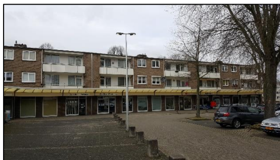
Figuur 1.19 Complex 1-0120-BR/Complex 1-0086-W1
