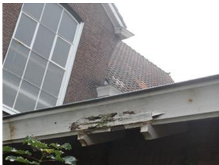
Gaten in bekisting
