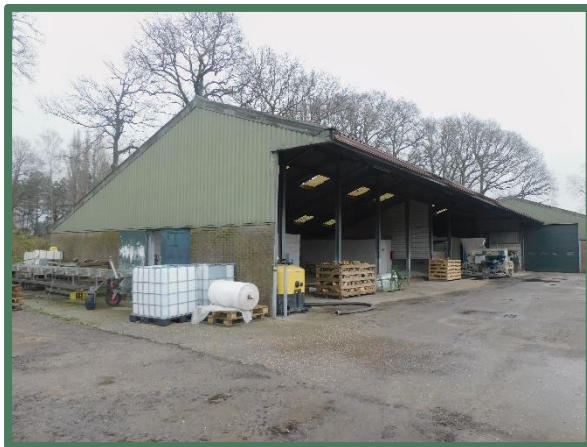
Te slopen open loods
