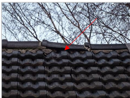
Foto 11: Impressie plangebied (openingen dak woning).
