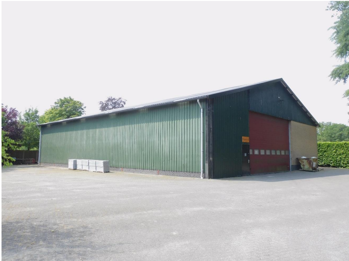
Te slopen loods
