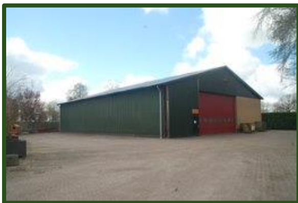
Te slopen loods
