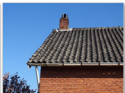
Foto 7: Dak van woning.
