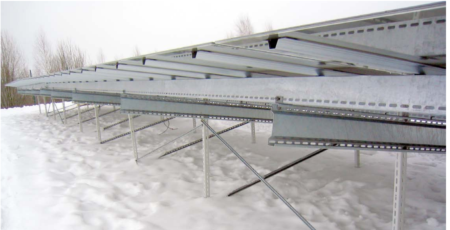
Modules, thin-film with back rails, 2.6 x 1.1 m, 2-rows, portrait
