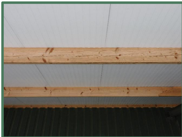
Damwandpanelen daken loods
