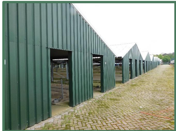
Damwandpanelen wanden stallen
