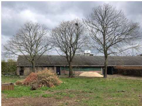
9. Te slopen stal
