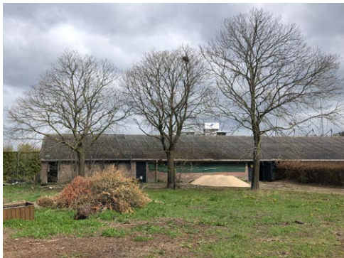
9. Te slopen stal
