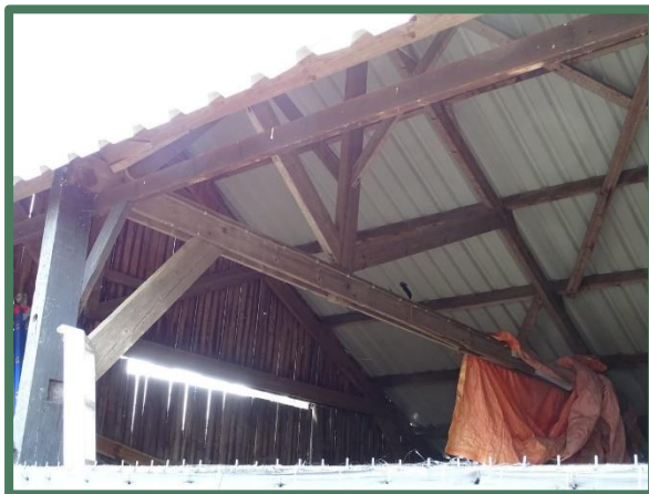
Damwand dak te slopen stal
