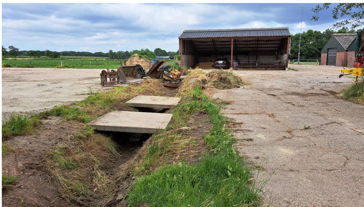
Depots achter caravanstalling (5)
