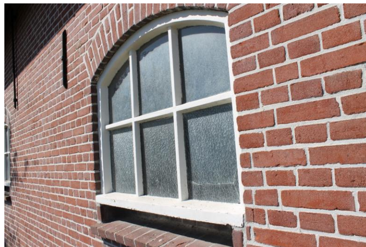
Later aangebrachte betonvensters.
