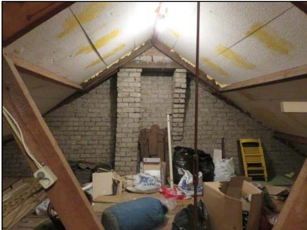
Foto 5. Zolder te slopen pand
