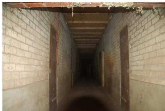
centrale gang stal 4
