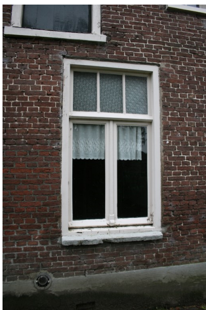
Later aangebracht venster
