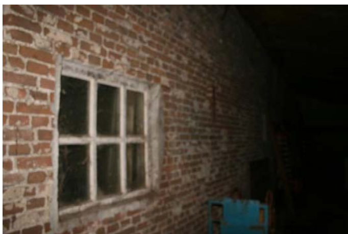
Later aangebracht betonnen stalraam
