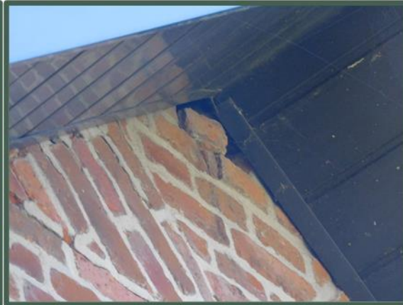
Opening in de nok
