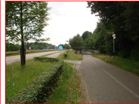
Start tunnelbak segment III
