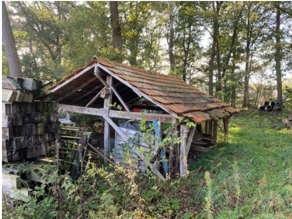
Te slopen kippenhok/houthok
