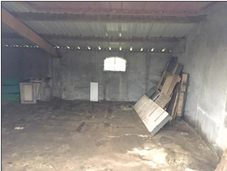
Berging (te slopen)
