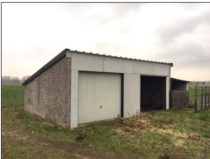
Berging (te slopen)
