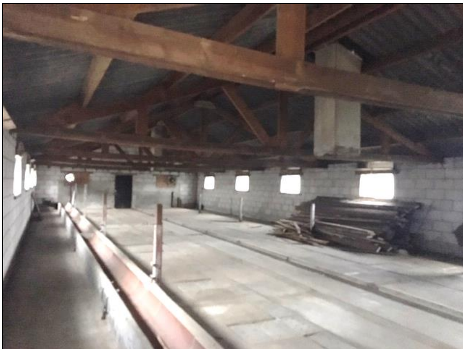
Stal 2 (te slopen)
