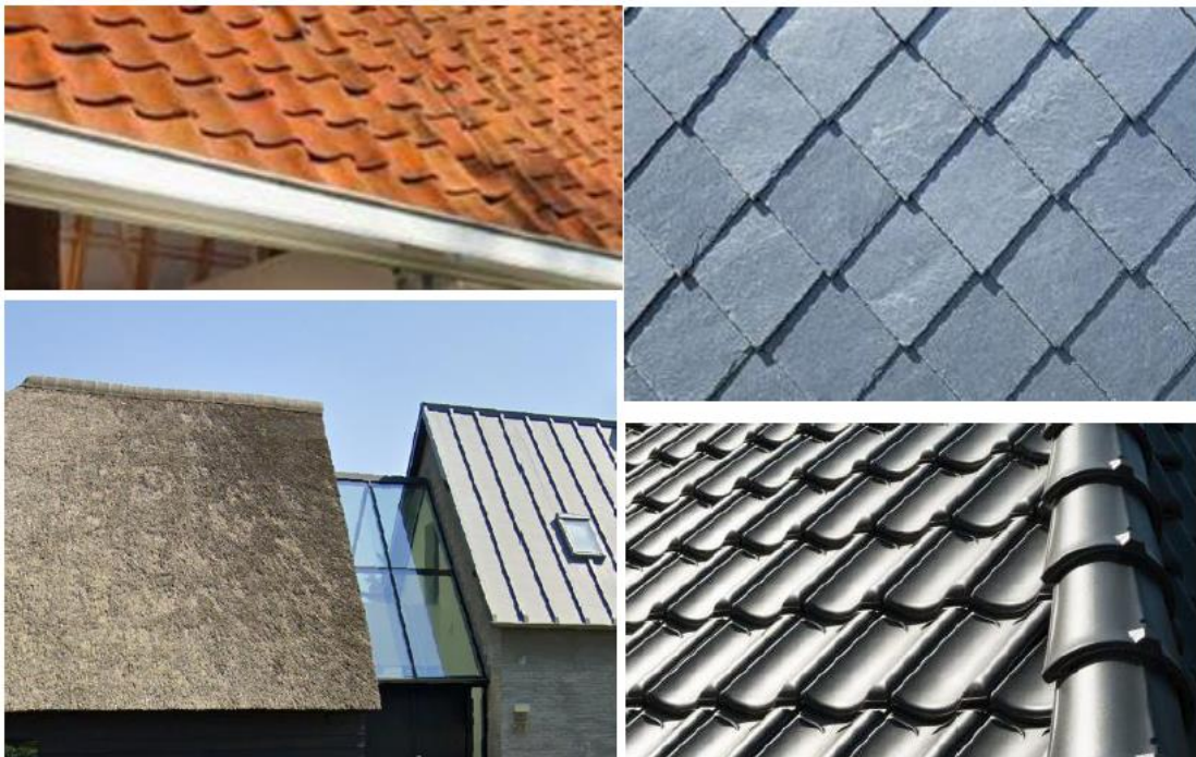
Figuur 16: referenties dakbedekking
