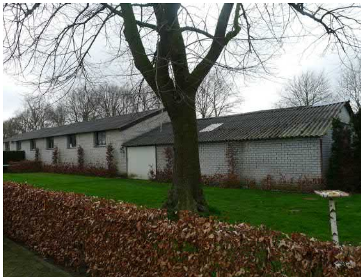
TE SLOPEN STAL
