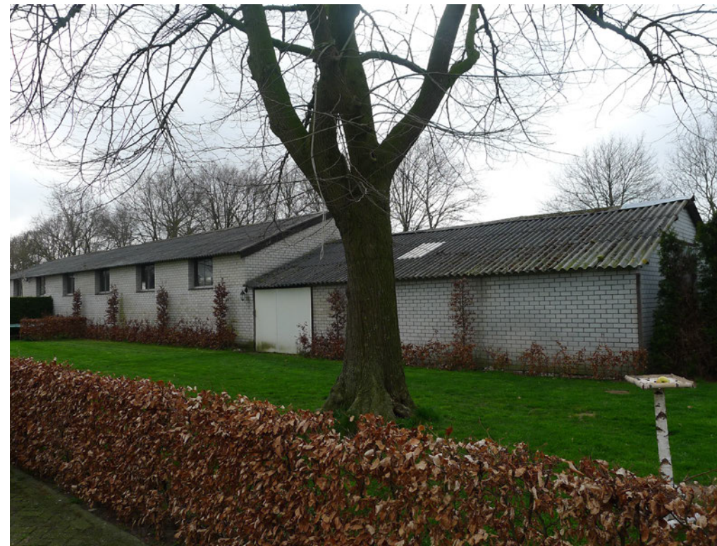
TE SLOPEN STAL
