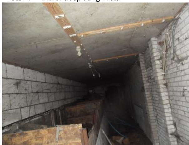
Foto 2: Plafondbeplating in stal
