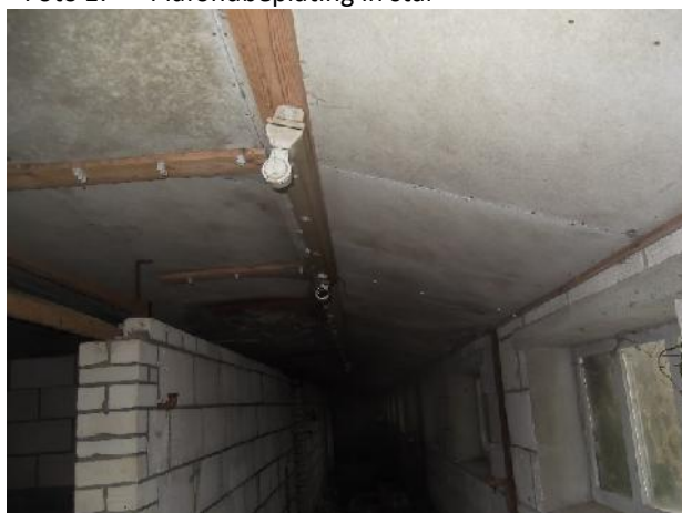
Foto 1: Plafondbeplating in stal
