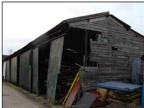
Foto 1. Te slopen loods
