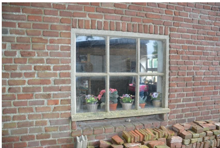
Detail venster in achtergevel.
