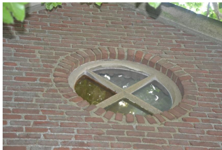
Detail oculus in achtergevel.
