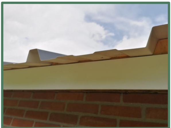
Sandwichpanelen dak garage
