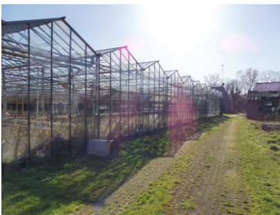
Te slopen kassencomplex.
