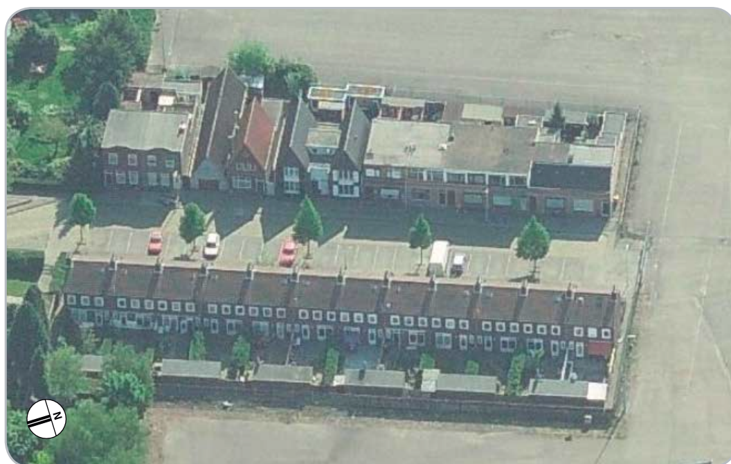
Gevelaanzichten (bron: bing.com/maps )
