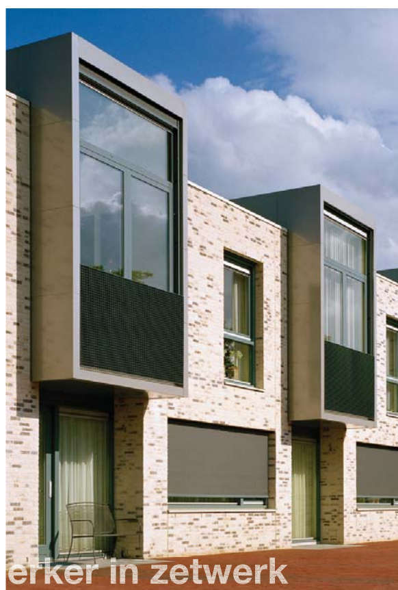
erker in zetwerk
