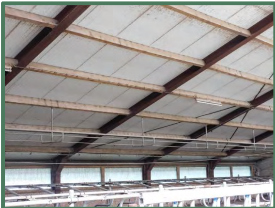
Sandwichpanelen dak rundveestal
