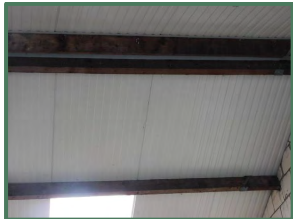
Sandwichpanelen dak te slopen loods
