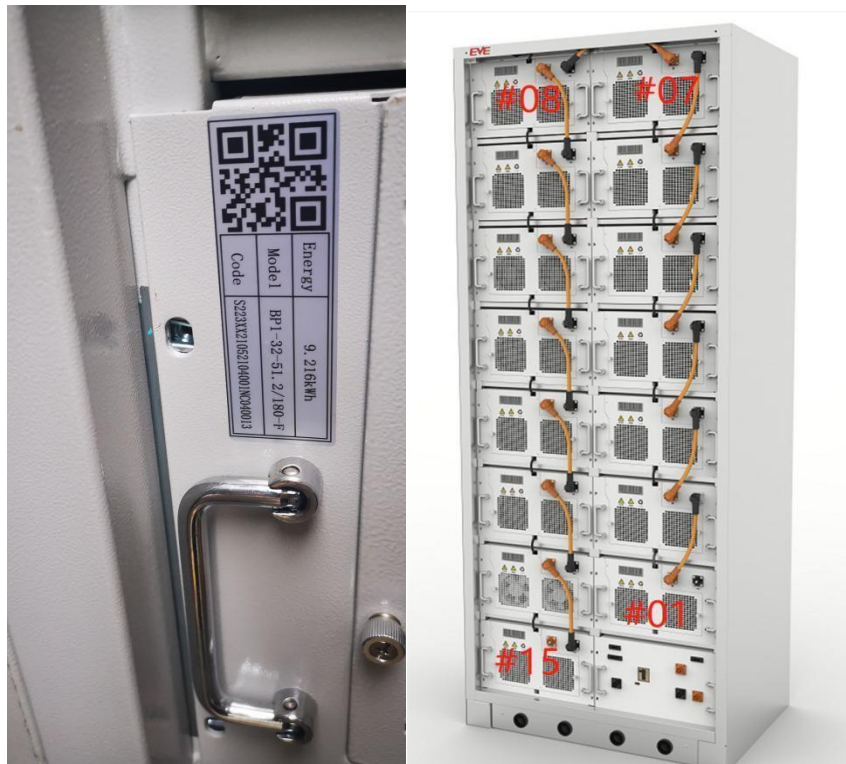
Figure5-2 Battery Installation Sequence
