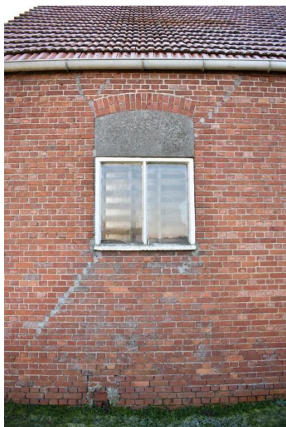
Later aangebracht betonvenster.
