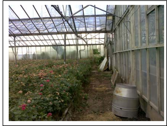
Foto 8: Toegang richting stookhok
