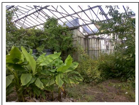
Foto 6: Basin tpv stookhok
