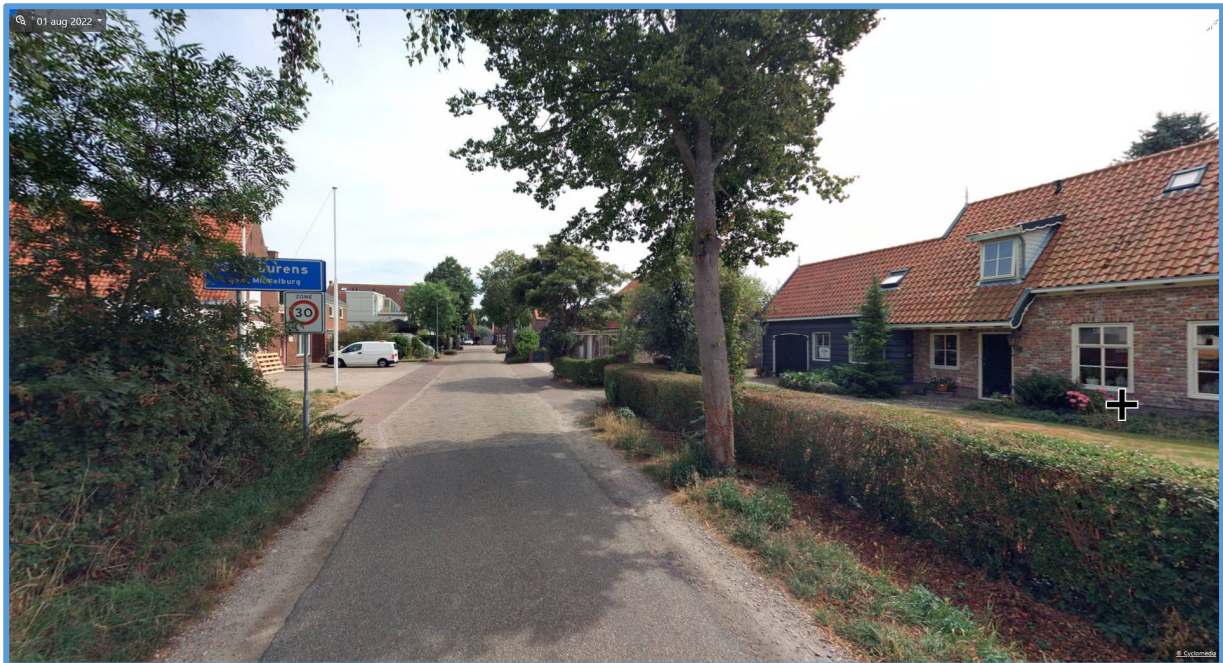
Figuur B (bron: https://streetsmart.cyclomedia.com/streetsmart )
