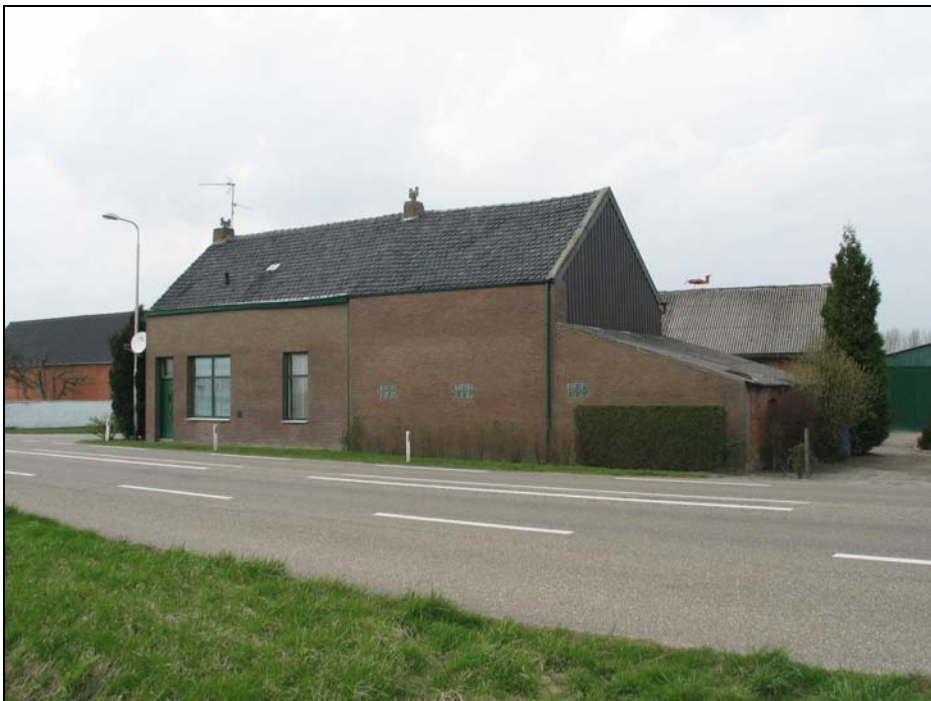
Foto 5 Te slopen woning
