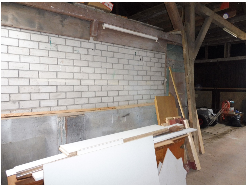
20: kalkzandsteen wand garages in de as van gebint 5
