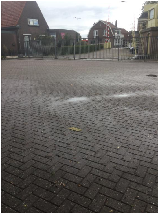
Foto 4: Boring 01 (d.d. 27 september 2022)
