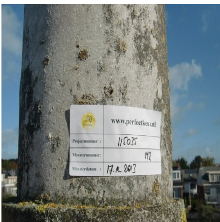
M2 is asbesthoudend.
