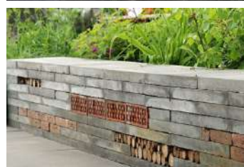
Muur/zit element Beton, porrobrick, hout Ecologisch interessant
