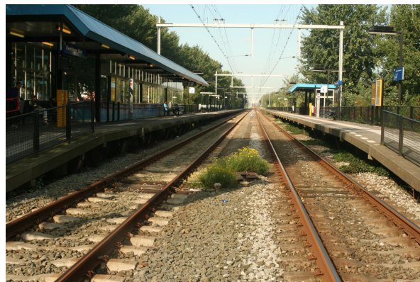
Figuur 4.14 Station Vlaardingen West.
