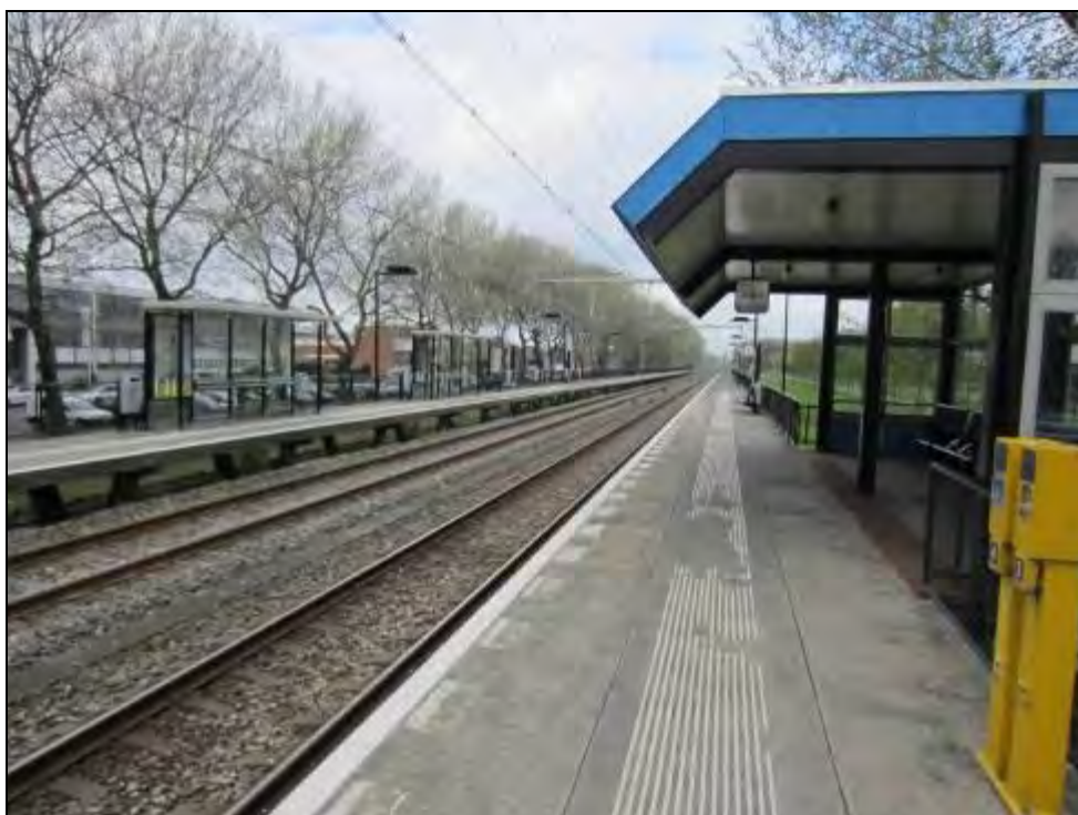
Figuur 5.5 Station Vlaardingen West
