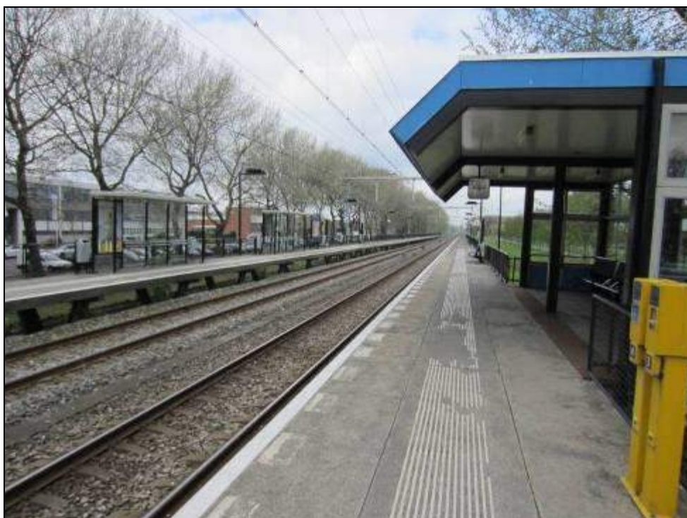
Figuur 5.5 Station Vlaardingen West
